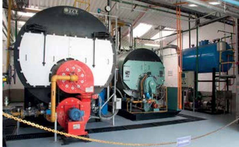
Changing fuel in boilers. The Cárnicos Nutresa Plant, La Ceja
