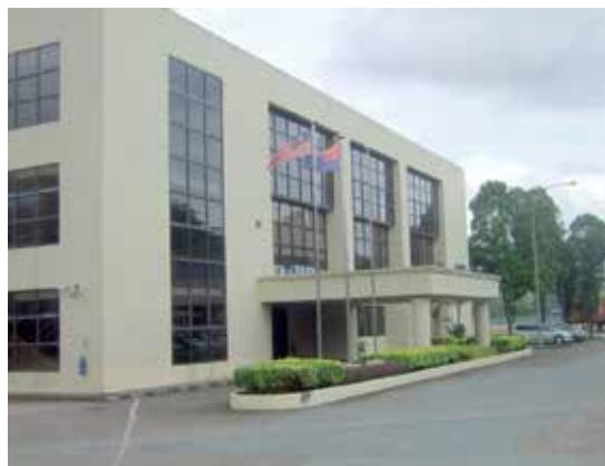
The DKM Headquarters, Malaysia
